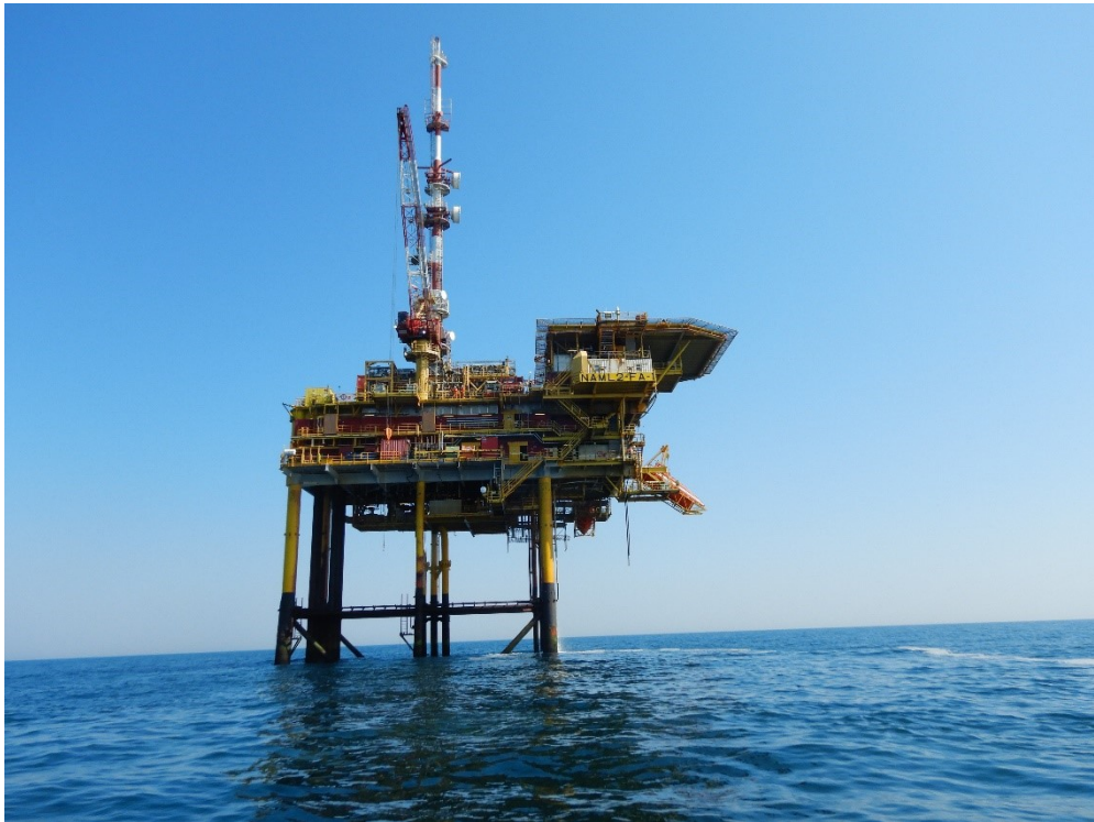
Figure 3.1: Tenaz Energy platform L2-FA-1
