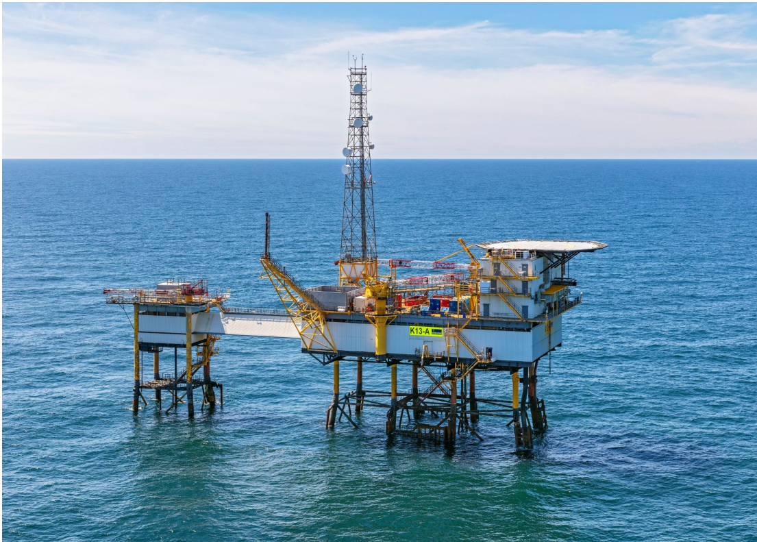
Figure 3.1: Wintershall platform K13-A
