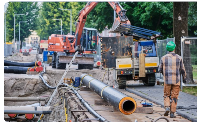
Construction of the heat grid
