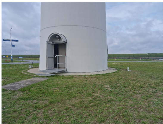
Figure 2.3: Picture of turbine 21 with two pairs of cameras mounted on either side
