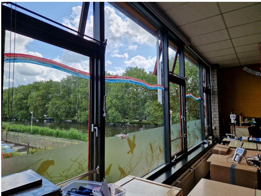
Figure 1-2 – Ventilation system before intervention
