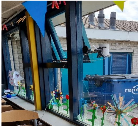
Figure 1-2 – Ventilation system before intervention
