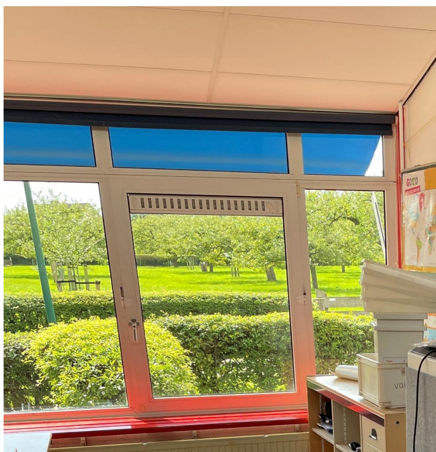
Figure 1-2 – Ventilation system before intervention
