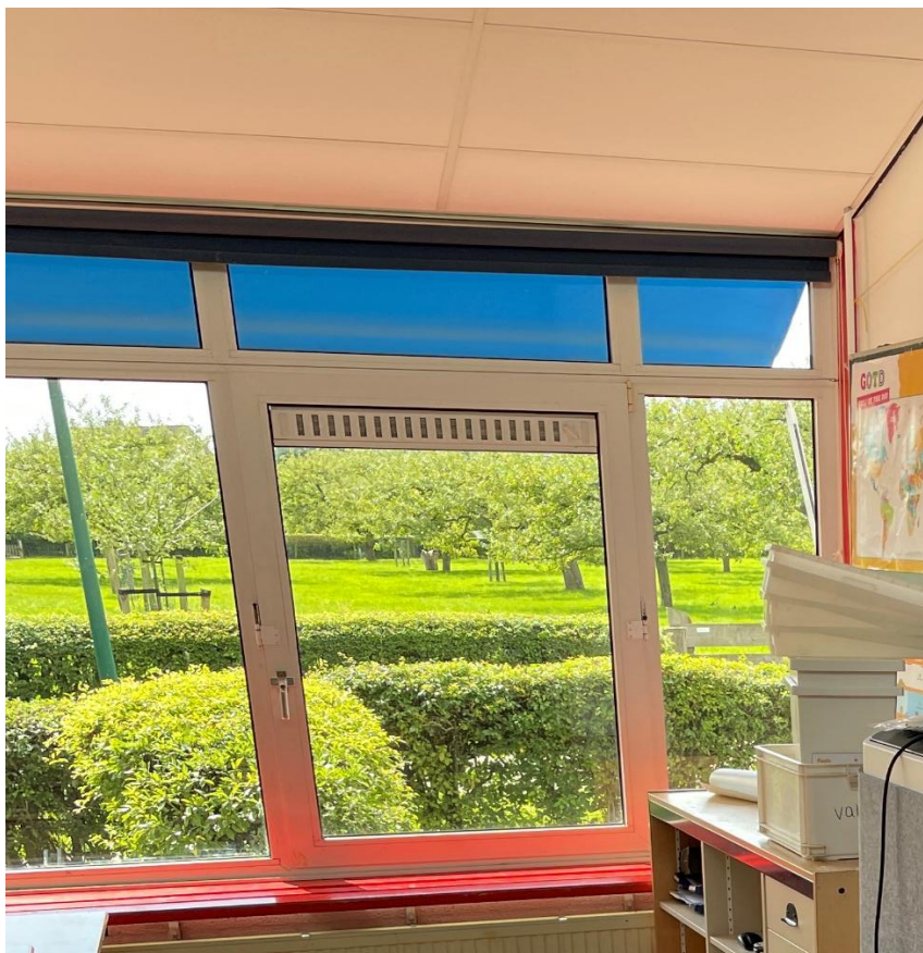
Figure 1-2 – Ventilation system before intervention
