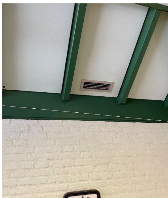
Figure 1-2 – Ventilation system before intervention
