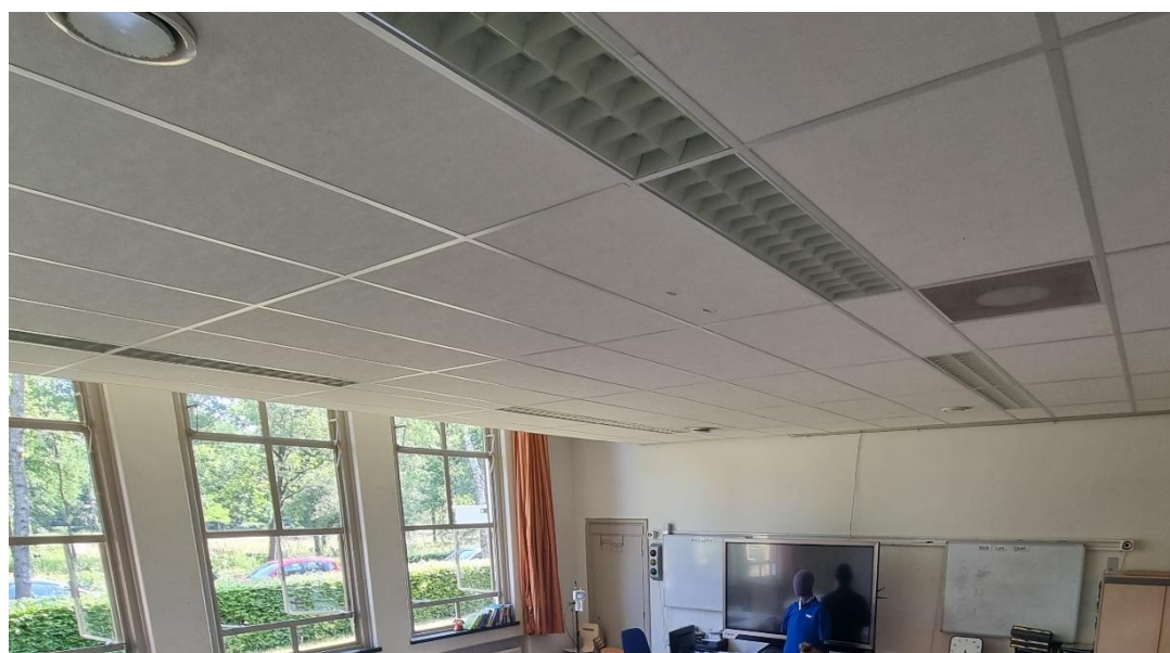
Figure 1-2 – Ventilation system before intervention
