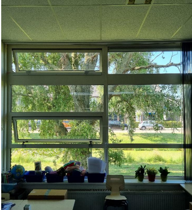
Figure 1-2 – Ventilation system before intervention
