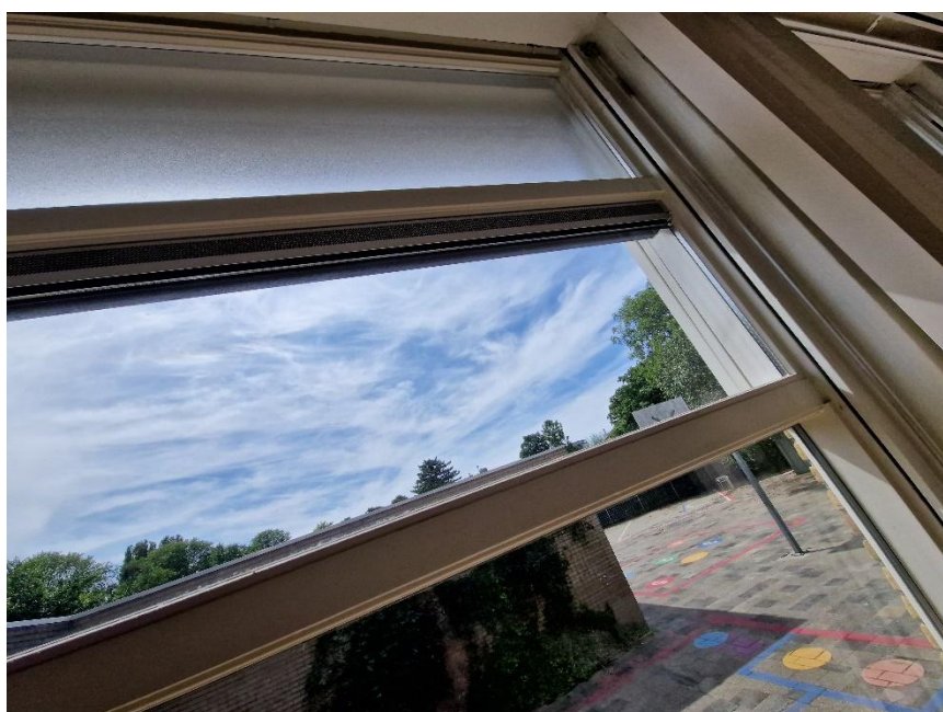
Figure 1.2 – Ventilation system before intervention
