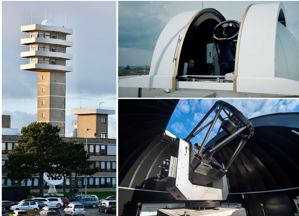
Figure 4. Pictures of the TNO OGS facility in The Hague, showing the tower with the dome on top (left), the opened dome (top right) and the ASA telescope inside the dome (bottom right).
