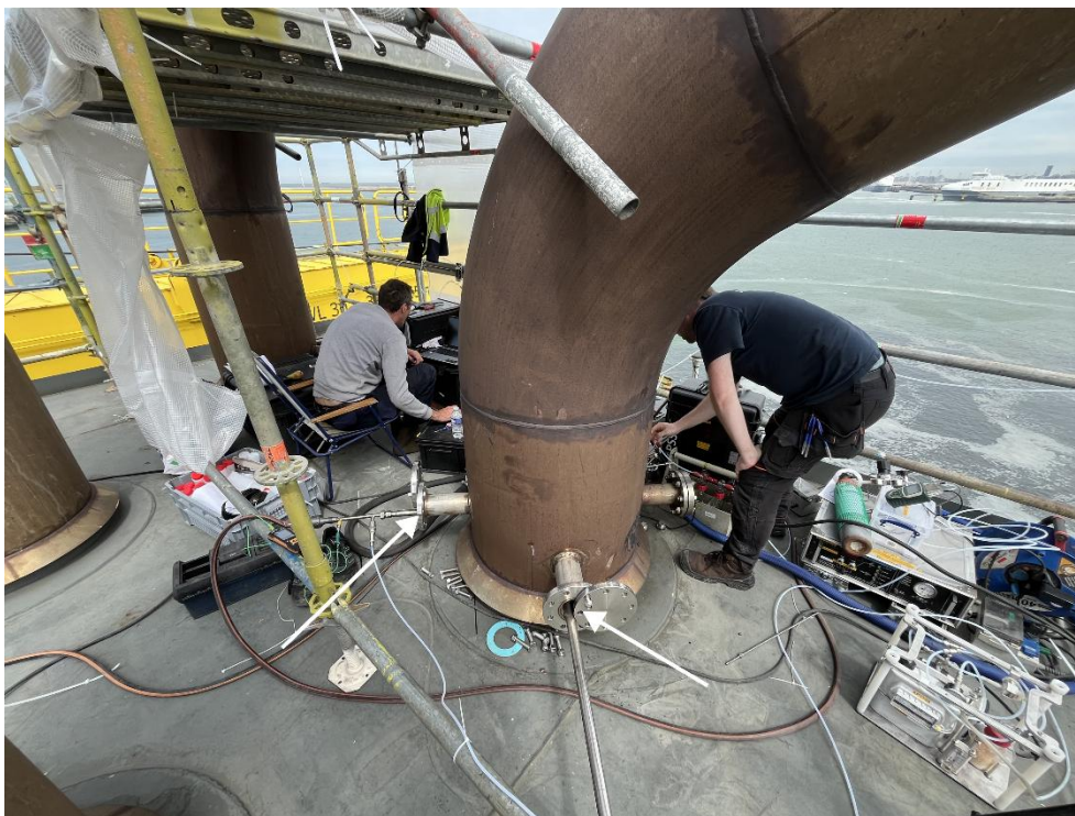
Figure 3.3: Sampling holes in the exhaust stack.
