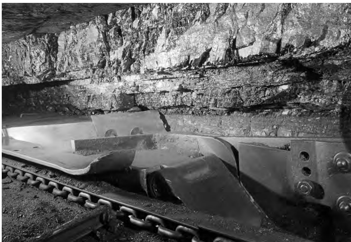
Figure 15.9. Mining equipment (kolenschaaf) in a pillar in the Oranje Nassau Mines taken around 1952. In the background a Westphalian coal seam is visible with the typical layering and break-out patterns of coal. © Nico Jesse / Nederlands Fotomuseum.
