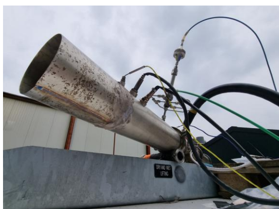
Figure 3.8: Exhaust Flow Meter (EFM) of the PEMS as mounted on the genset.
