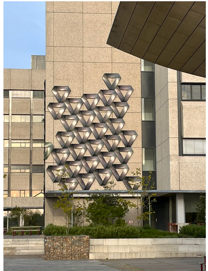
Fig. 8. East side of the building in the morning light, showing special visual effects due to the curvature of the elements.
