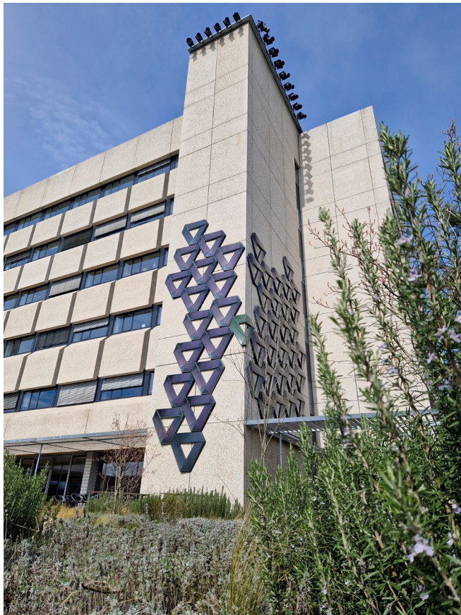
Fig. 7. Facade elements with PV after installation. South façade on the left with 15 elements; East façade on the right with 29 elements.
