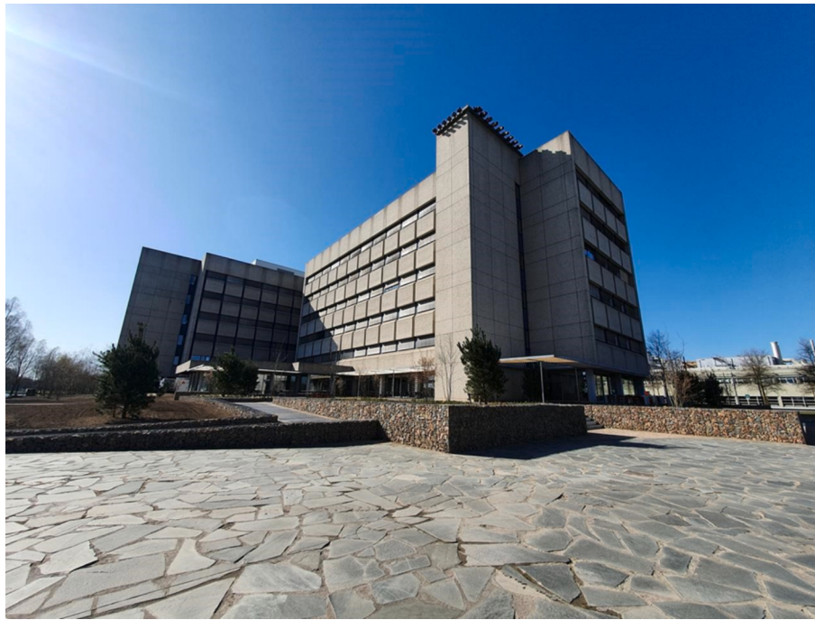
Fig. 1. Office building HTC 5 prior to the installation of the PV façade elements.
