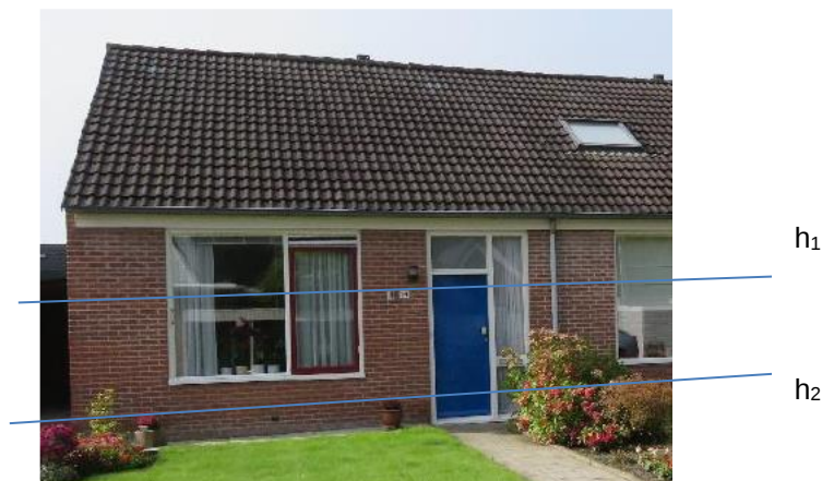
Figuur 7: Bepaling van percentage openingen in langsgevel.
