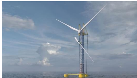
Figure 3.6: Blade installation/repair using the WindSpider crane technology
