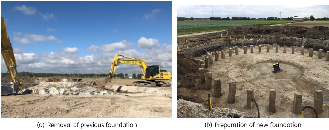
Figure 3.4: Illustration of turbine foundation works
