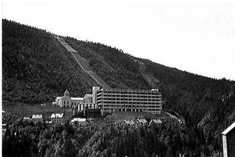
Figure 4 Vemork hydroelectric power plant in 1935 with H 2 production plant (front building)
