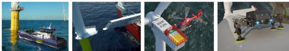
Figure 3. Access to the boat landing, TP platform landing, helideck/hoisting platform and autonomous inspection (from left to right)
