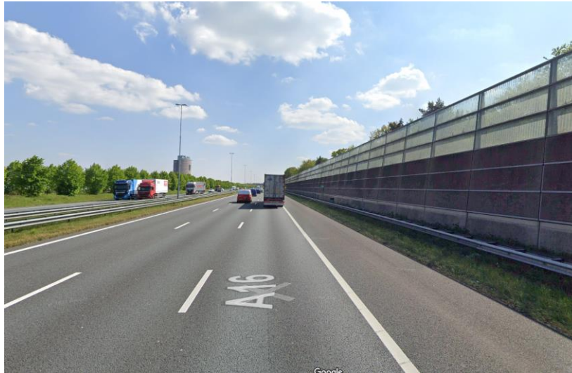
Figure 2-31. Frequent CACC dropout zone according to test drivers (potentially due to large barrier; image from Google Streetview).
