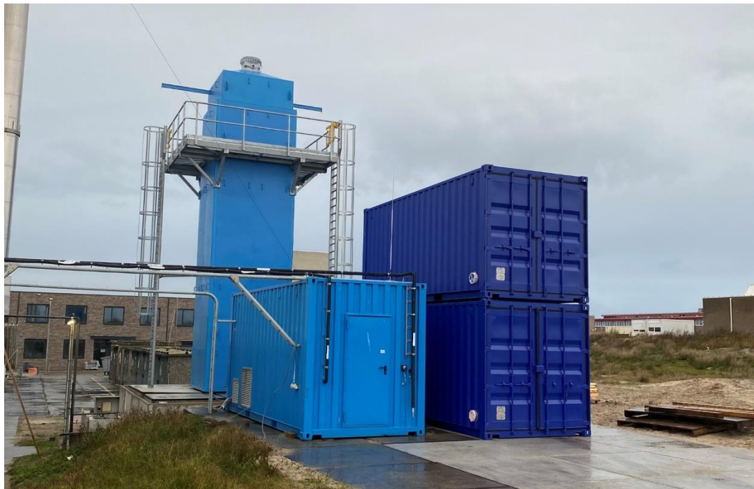
Figure 3: Nextgen container (left bottom container), and SEDMES unit in FLIE Petten.
