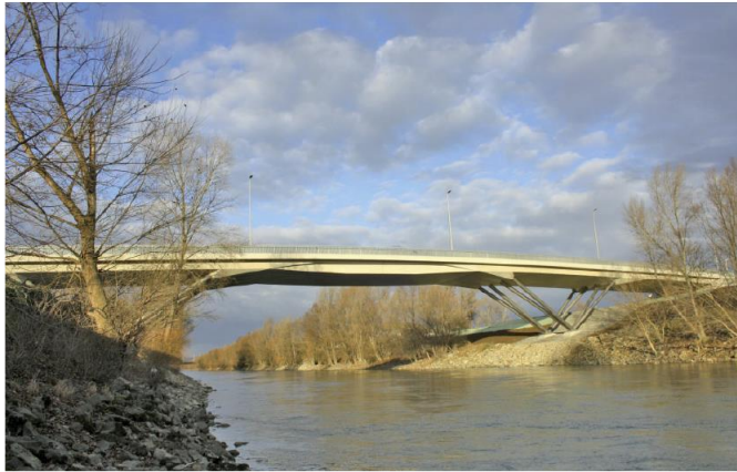
Figure 4 View of the Seitenhafenbridge, Vienna Austria
