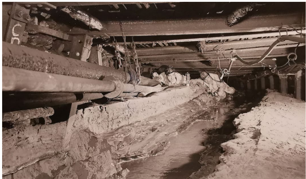
Figure 2: Two mineworkers inspect a mining gallery that was filled by an uncontrolled influx of quicksand and water. UD's were used to prevent this by allowing a manageable influx of quicksand. Mining gallery heights are in the order of >2 m, through which the 2 mineworkers are only able to crawl now.
