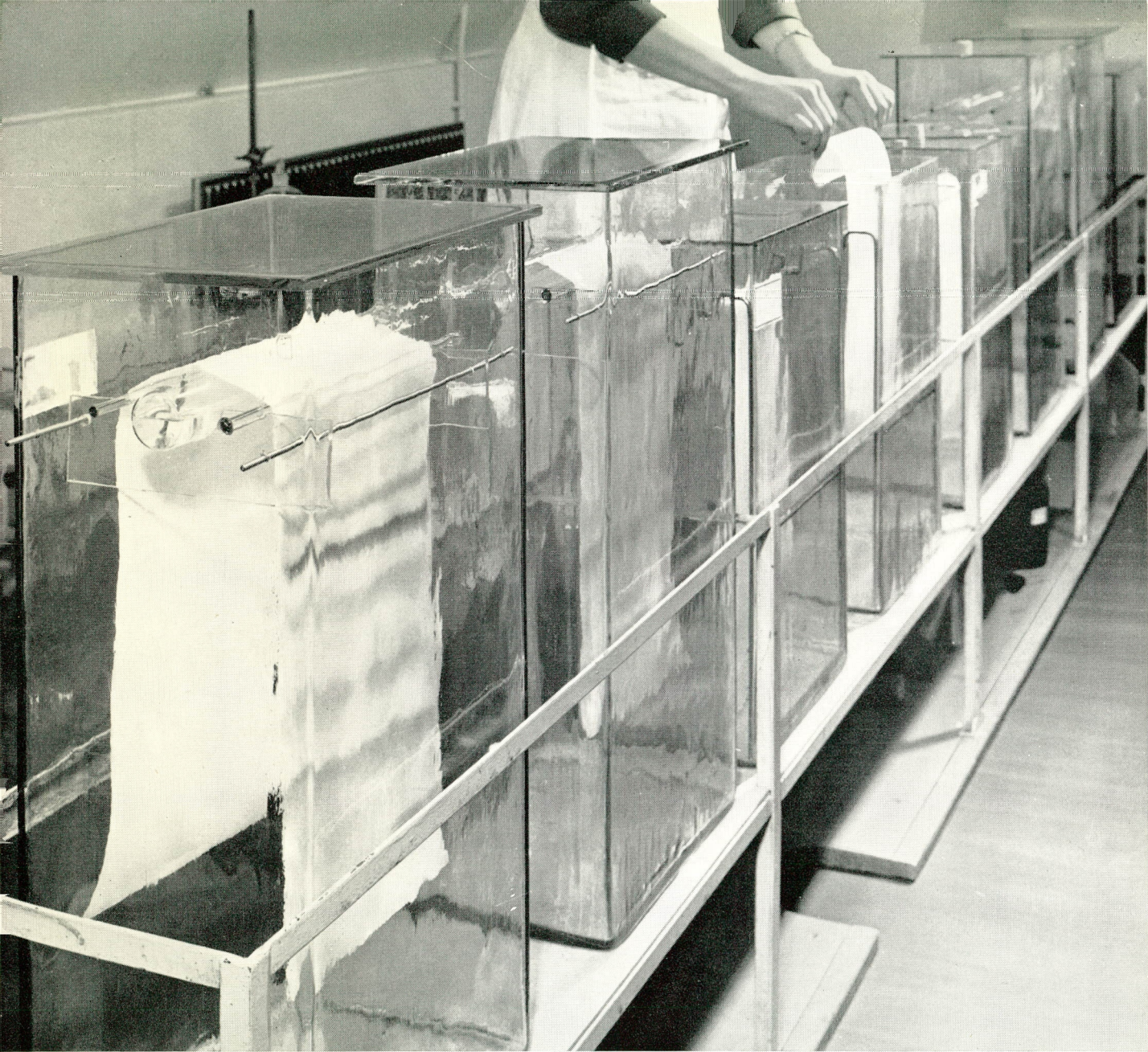
Tanks for paper chromatography
