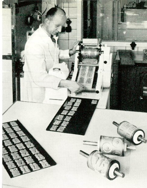
Biscuit cutting and moulding machine
