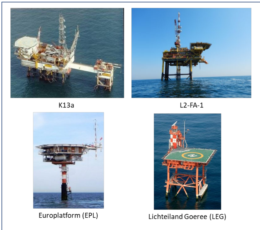
Figure 2.1 TNO offshore measurement platforms
