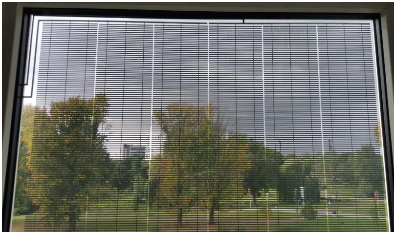
Figure 19: IGU with transparency achieved by using small c-Si PV cell-strips. © Pilkington Sunplus™ BIPV [20]
