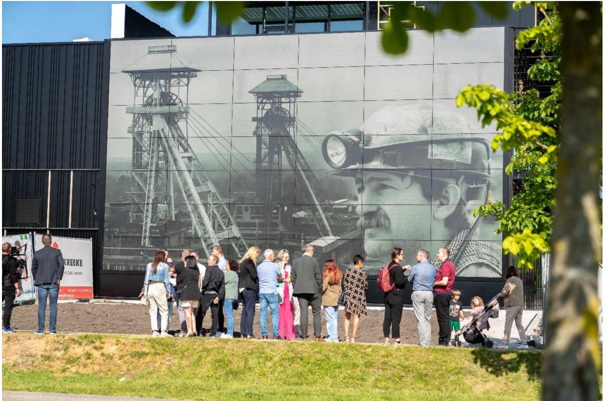
Facade of new R&D and production facility of SolarEMR-member Soltech is PV-active, and a very nice example of BIPV. 42 Patterned PV-panels form one total image which makes the integrated PV truly invisible!
