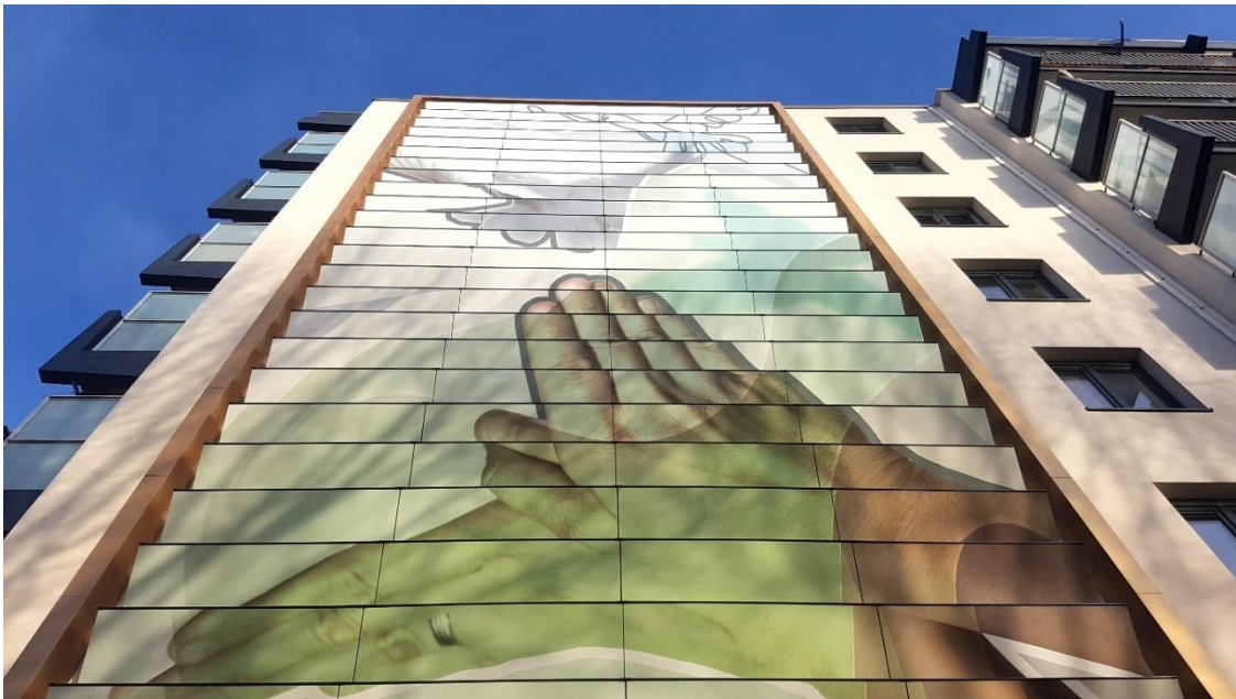
Figure 11: ZigZag solar has a regular product that is already custom-made with respect to the color and patterns on the downward facing parts of the facade. The PV-panels are integrated in the upward facing part and therefore invisible from ground level.
