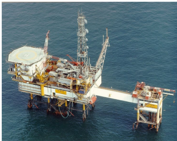
Figure 2: View of the K13a platform during visiting in November 2022 (left), location of K13a in the Dutch North Sea (right)
