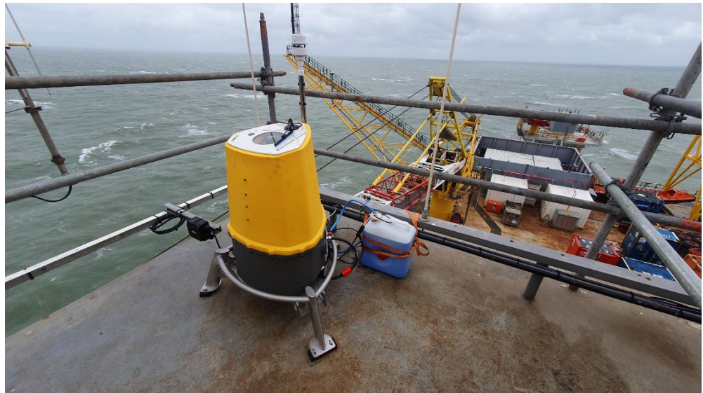
Figure 3: View of LiDAR unit following replacement in November 2022
