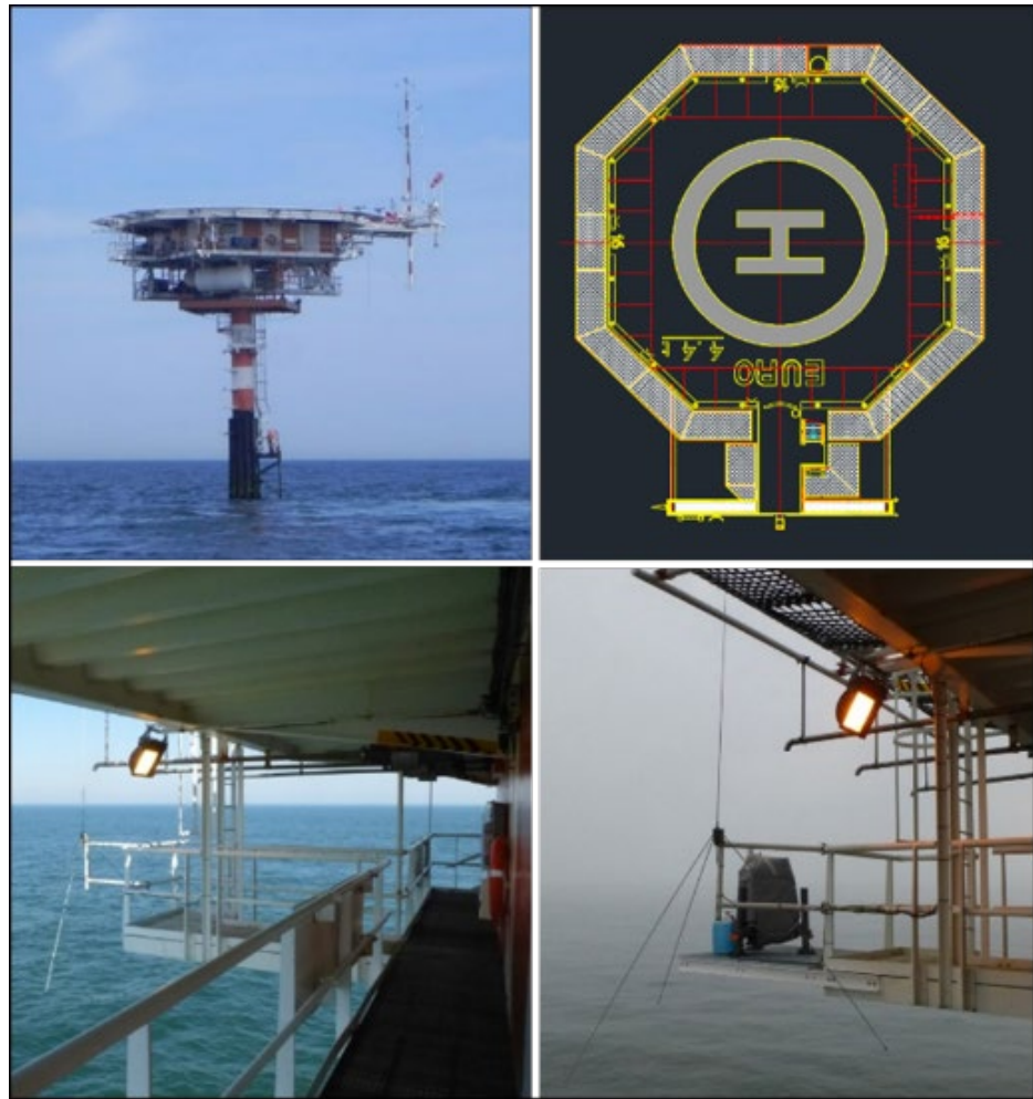
Figure 4: a) Front and b) top view of EPL platform (geographical coordinates 51° 59' 52.512" N, 3° 16' 29.316" E) including a helicopter deck at a height of 18.78m above mean sea level with an accommodation deck below; c) original escape ladder location before the LiDAR installation and d) built extension to install the LiDAR.
