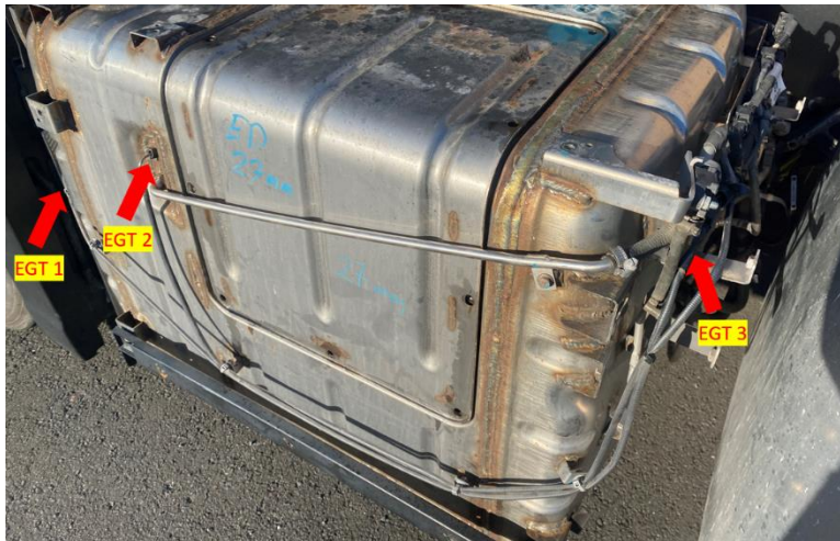
Figure 4.5: EPS unit with highlighted EGT sensors: EGT1 (before DOC), EGT2 (after DOC, before DPF) and EGT3 (before SCR, after DPF)
