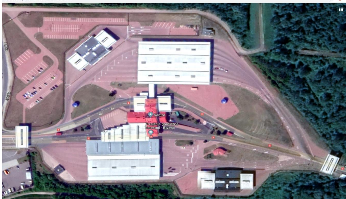
FIGURE 5-2.AERIAL VIEW OF BORDER CROSSING POINT IN TERESPOL
