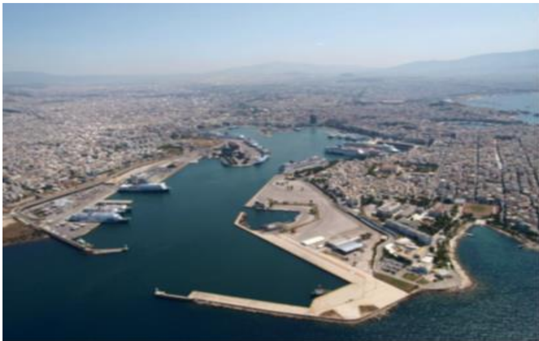
FIGURE 6-1. AERIAL VIEW OF THE CENTRAL PORT OF PIRAEUS
