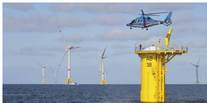
Figure 11: Offshore wind helicopter access.
