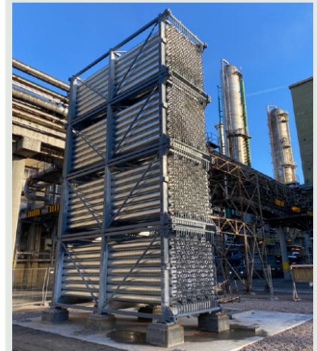
Figure 11 Four module ThermalBattery™ before insulation and cladding, during assembly at site in Norway [31].
