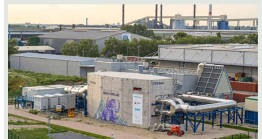
Figure 14 SIEMENS Gamesa's Carnot-battery thermal storage pilot plant in Hamburg [35].
