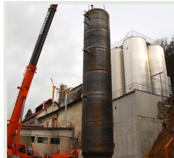
Figure 7 Solar-water TES in Hofmühl Brewery, Germany [26].
