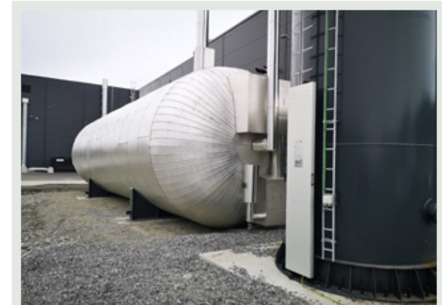
Figure 10 Steam accumulator (175 m 3 ) implemented at a large poultry processing plant in Orkanger, Norway [30].
