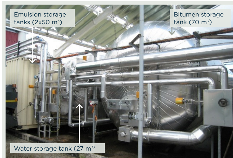
Figure 8 Emulsion, bitumen and water storage tanks in Colas, Switzerland SA [22, 27].
