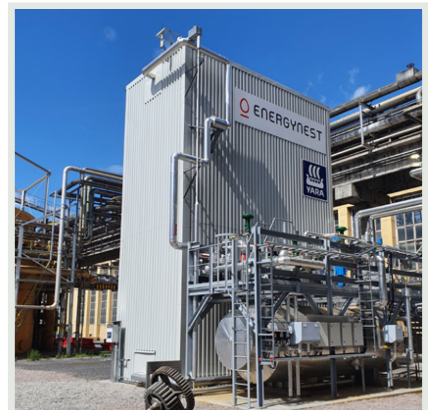
Thermal storage battery, Herøya, Norway.
