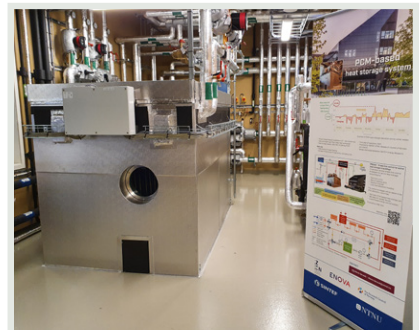
PCM-based heat storage system at the SINTEF/NTNU ZEB Laboratory, Trondheim, Norway.
