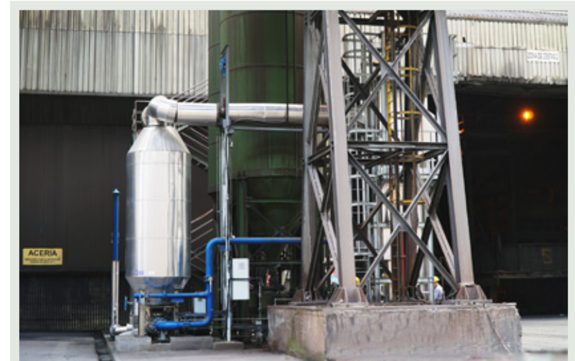
Figure 6 CIC EnergiGune packed bed TES at the ArcelorMittal steel recycling plant [23, 24].
