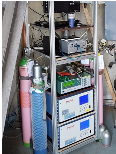
Figure 2 Measurement instruments in the tower.
