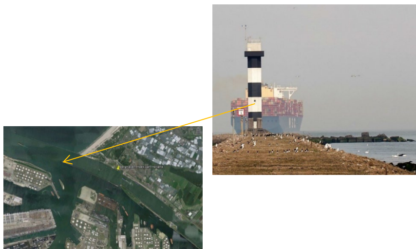
Figure 1 The tower and its location on the map at the port of Rotterdam.
