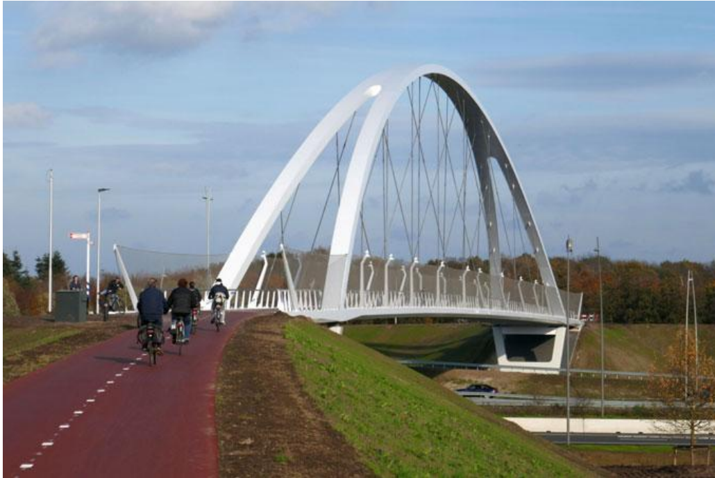
Fig. 1 Bicycle bridge Tegenbosch [13]
