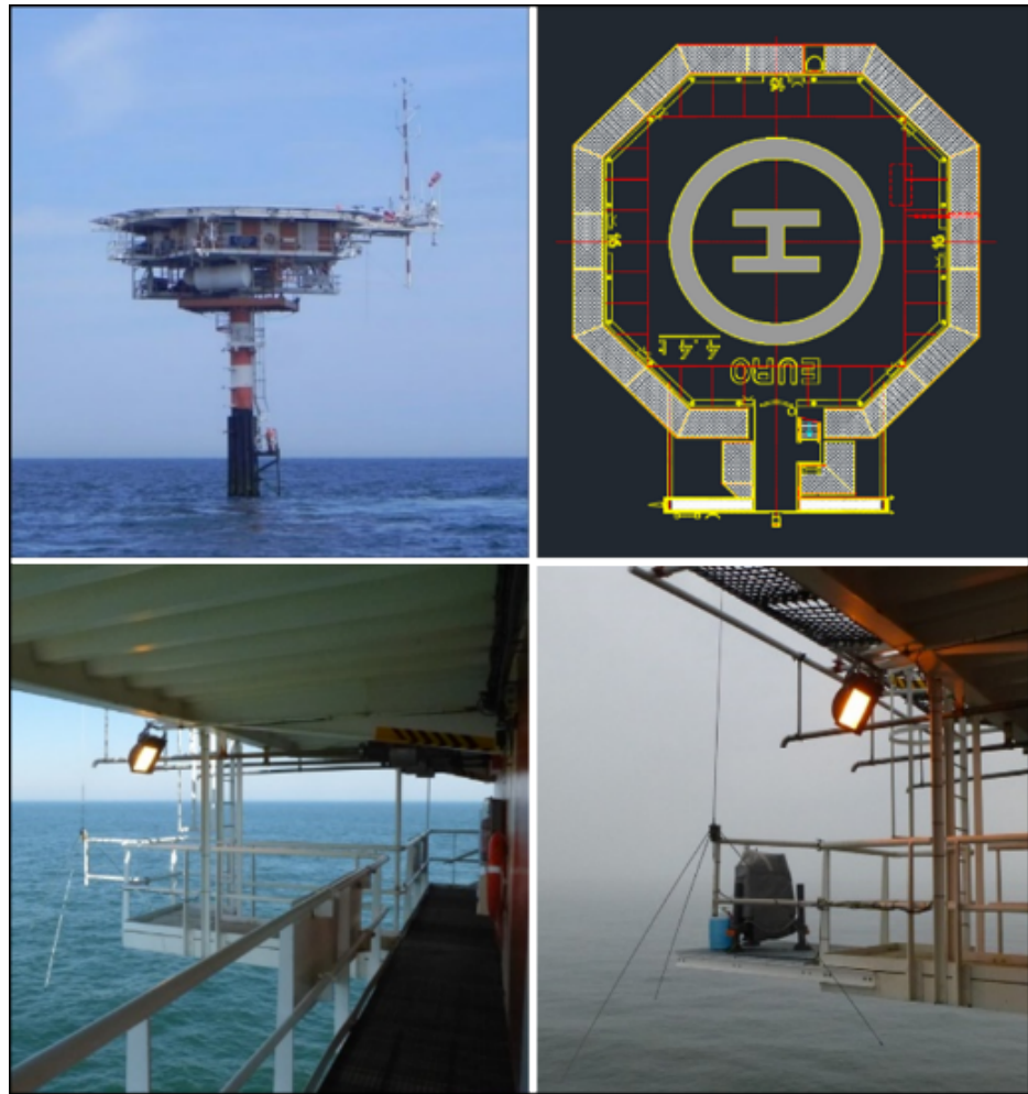
Figure 6 a) Front and b) top view of EPL platform (geographical coordinates 51° 59' 52.512" N, 3° 16' 29.316" E) including a helicopter deck at a height of 18.78m above mean sea level with an accommodation deck below; c) original escape ladder location before the LiDAR installation and d) newly built extension to install the LiDAR
