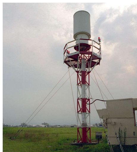
a. A US Air Force TACAN antenna, from [4]
