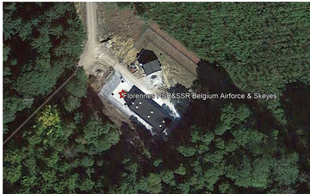
Figure 2.3 The Airport Surveillance Radar at Florennes Military Airbase, still under construction (image: Google Earth).
