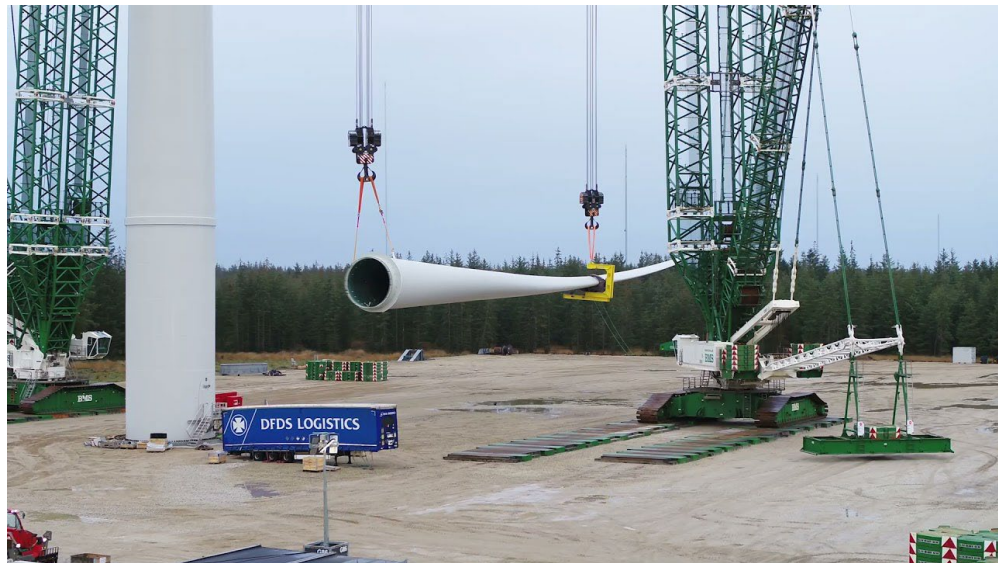
Figure 3-8 Two-crane SG14-222dd blade installation (source: still from https://www.youtube.com/watch?v=zoAOIrdT46g )
