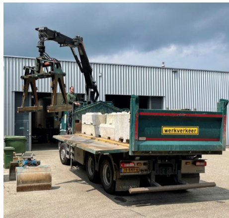
Figure 3-4: Using the PTO propelled hydraulic crane to unload concrete blocks from the vehicle.
