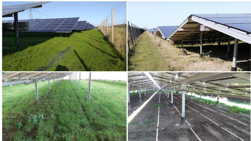
Figure 1 Left South oriented configuration with ample vegetation below panels and right east-west orientation deprived of vegetation below panels. Photo: Alex Schotman WUR
