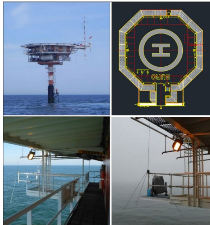
Figure 3 a) Front and b) top view of Europlatform platform (geographical coordinates 51° 59' 52.512" N, 3° 16' 29.316" E) including a helicopter deck at a height of 18.78m above mean sea level with an accommodation deck below; c) original escape ladder location before the LiDAR installation and d) newly built extension to install the LiDAR.
