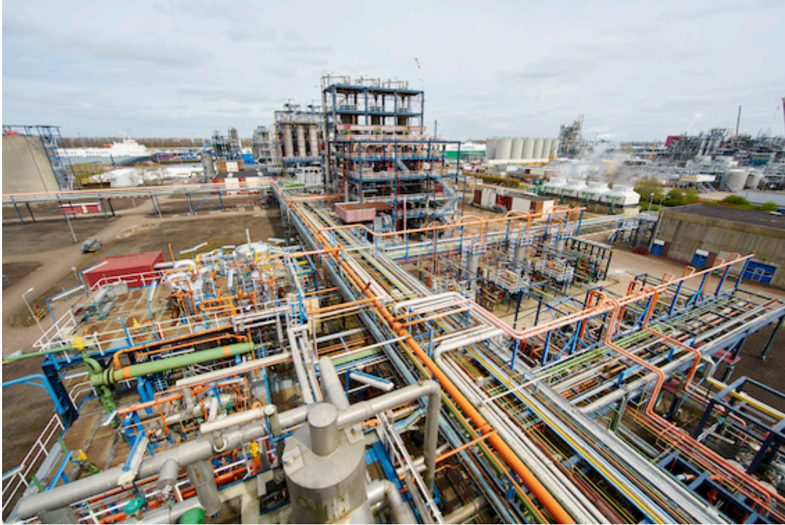
Figure 4 View of Ducor chemical plants in the Rozenburg site (Ducor, 2020b).
