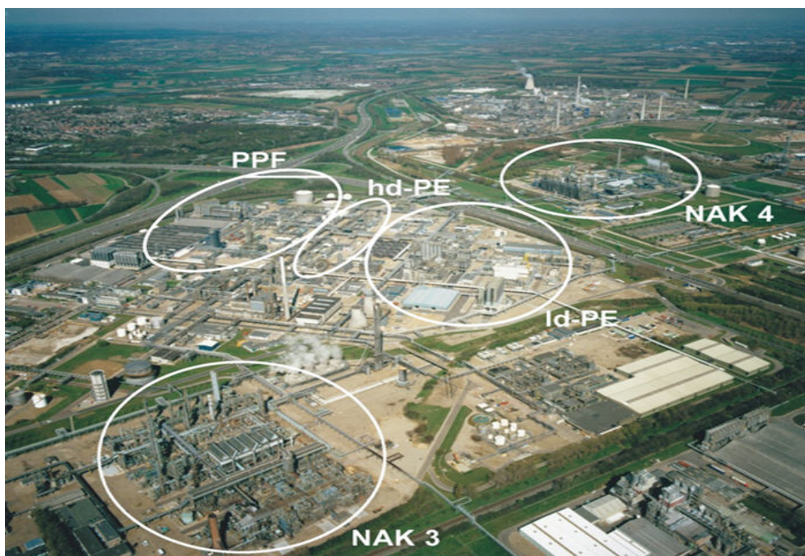
Figure 3 Aerial view of SABIC chemical plants at Chemelot industrial park, showing the naphtha crackers NAK3 and NAK4, and the production lines of PP, HDPE and LDPE (SABIC Limburg, 2020).
