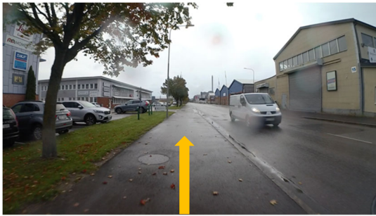
Figure 10-17: The lane edge to the right acts as an insufficient divider. Cyclists travel in the middle of lane.
