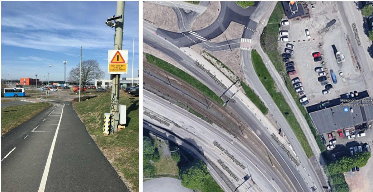
Figure 10-2: Site 2. The installed nudge (left), note the Viscando Otis measuring equipment mounted on the light pole nearest in the picture. The Götaälvbron site (57°43'12.4"N 11°57'45.5"E), the bike lane is the lane most to the right in picture (right).
