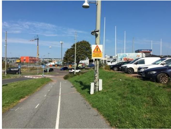
Figure 10.5: The equipment installed at one of the locations (Götaälvbron).
