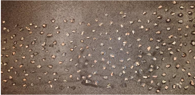
Figure 8-2. Gravel on roofing felt.
