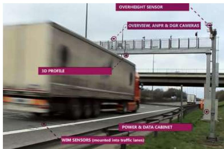
Figure 5.4: High speed WIM systems for load measurements, licence plate recognition (video) and 3D-profile scanning (reference [sterela-its.com](http://sterela-its.com))
