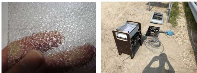
Figure 3 Left: cover material to give protection to PV and avoid reflections; Right: invertors to be placed below ground for safety reasons
