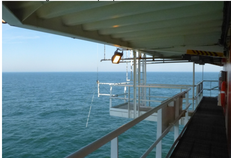
Figure 6 Extension of accommodation deck
