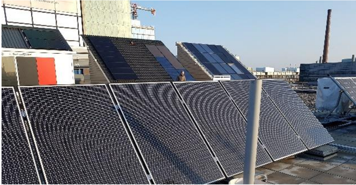
Figure 26. Picture of the TESSERA system. A pole is casting shade on several modules
