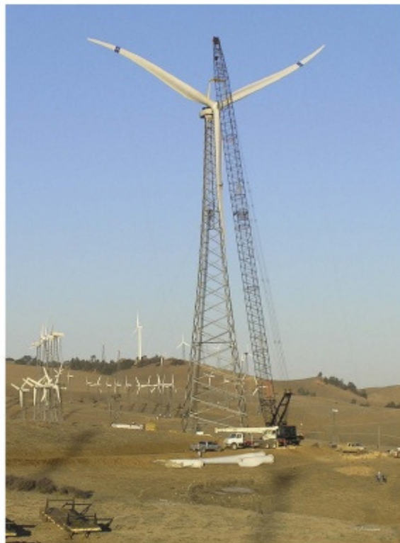
Sweep-twist adaptive rotor (STAR) prototypes were installed on a Zond 750 kW turbine at the TerraGen wind site in Tehachapi, California. Of note are the aft sweep of the tip and the trailing edge curvature. MD Zuteck
