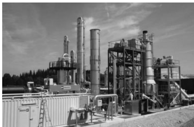
Figure 16. 1.1 MW e PRMe gasifier with OLGA in France.
