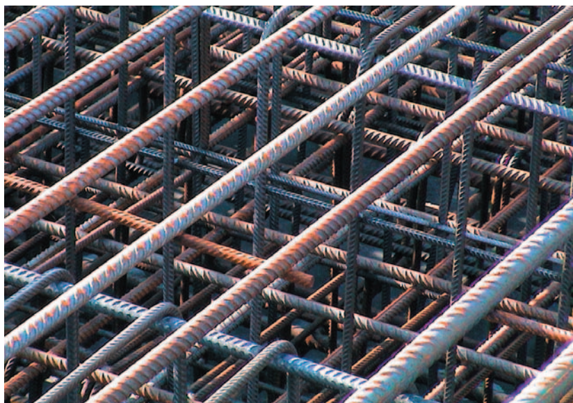
Additional strengthening for the foundations of the WMC complex.
