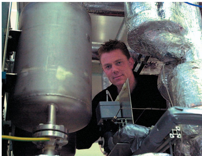
A Fuel Processor test installation is taken into operation. This installation is able to convert fuels into Hydrogen on a 50 kWe scale. On the picture BCT-employee Wilko Planje.
