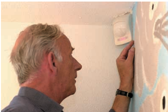
Jan Römer shows the occupancy detector that combines with the water meter in the alarm system.
