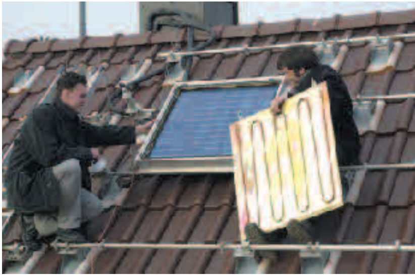
Marcel Elswijk en Herbert Zondag are mounting two specimens of a prototype of a solar panel (for electricity) and a solar collector (for heat) combination. Nearly all the energy from the sunlight can thus be utilised.
